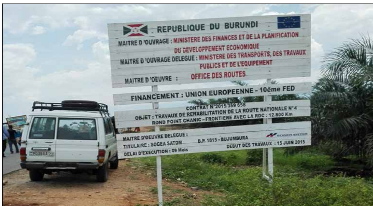
Photo: Bujumbura-Gatumba Road which is under construction with EU financial support
