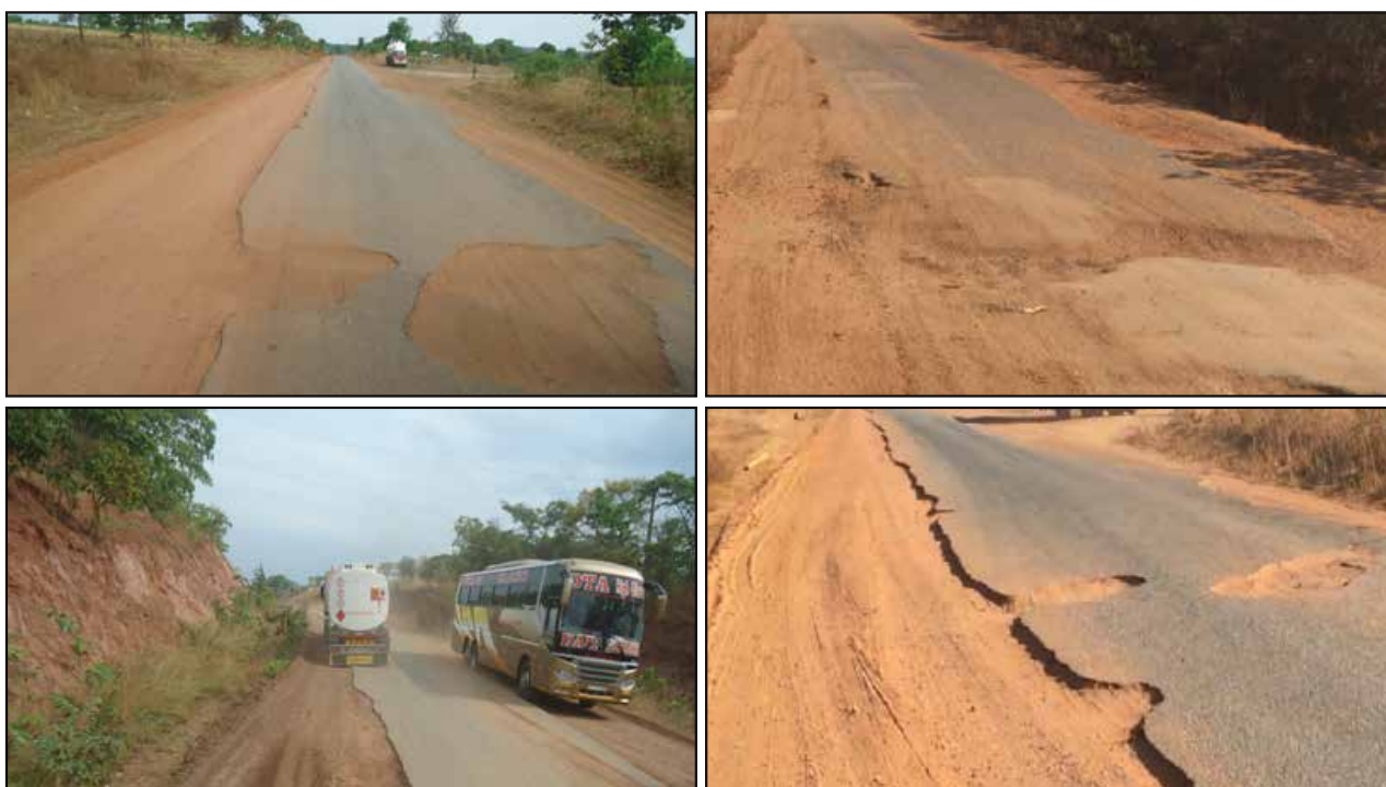
Photo: POOR ROAD CONDITION: Road section of Nyakanazi – Rusahunga Junction – Rusumo is in a poor condition with a large number of big holes and rough dust condition. The situation becomes worse during rainy season accidents and theft were reported at this main section of the central corridor roads.
