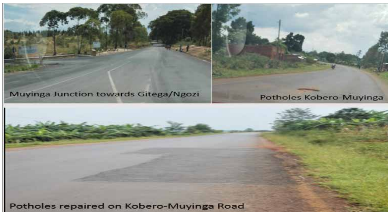
Photo: Kobero-Bujumbura road, 95% is in good condition despite some sections with potholes
