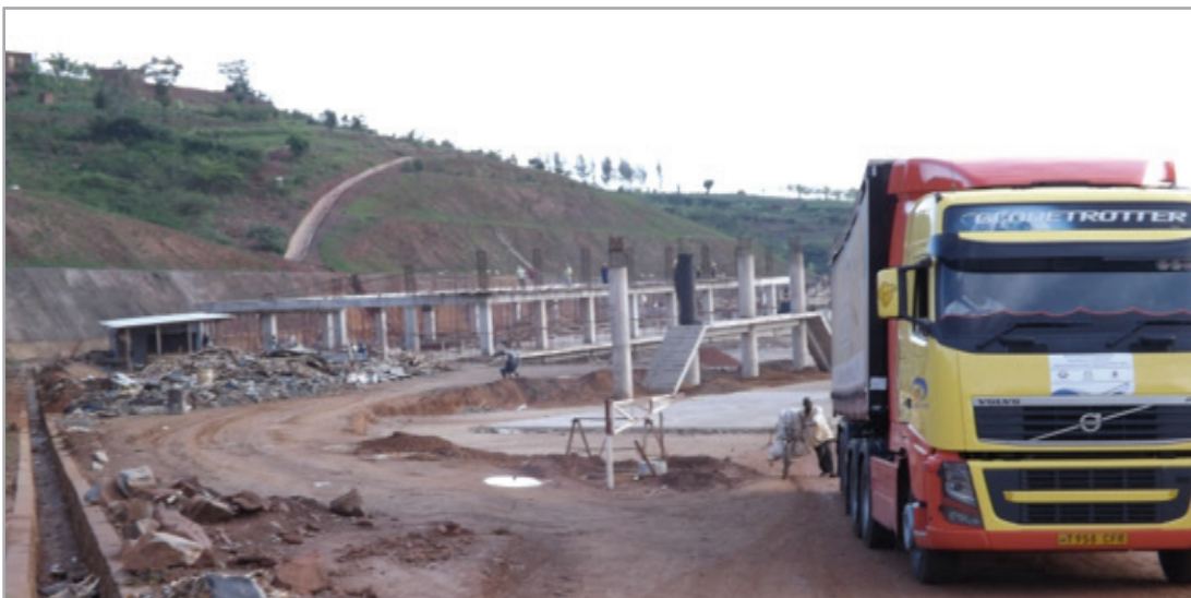
Rusumo border post under construction
