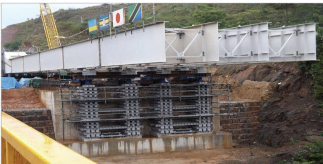
Rusumo bridge under construction
