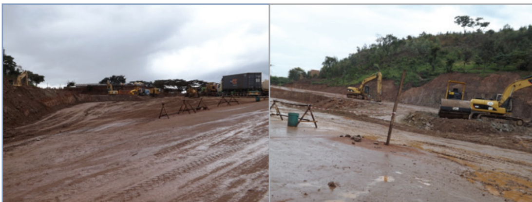
Rusumo border post under construction
