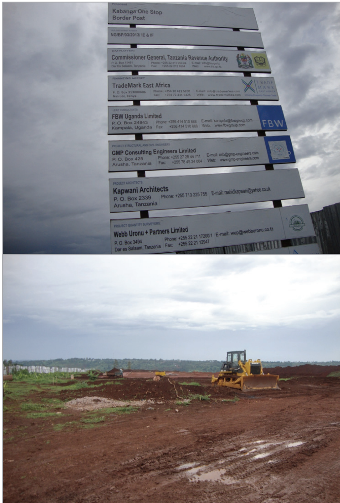
New Kabanga border post under construction
